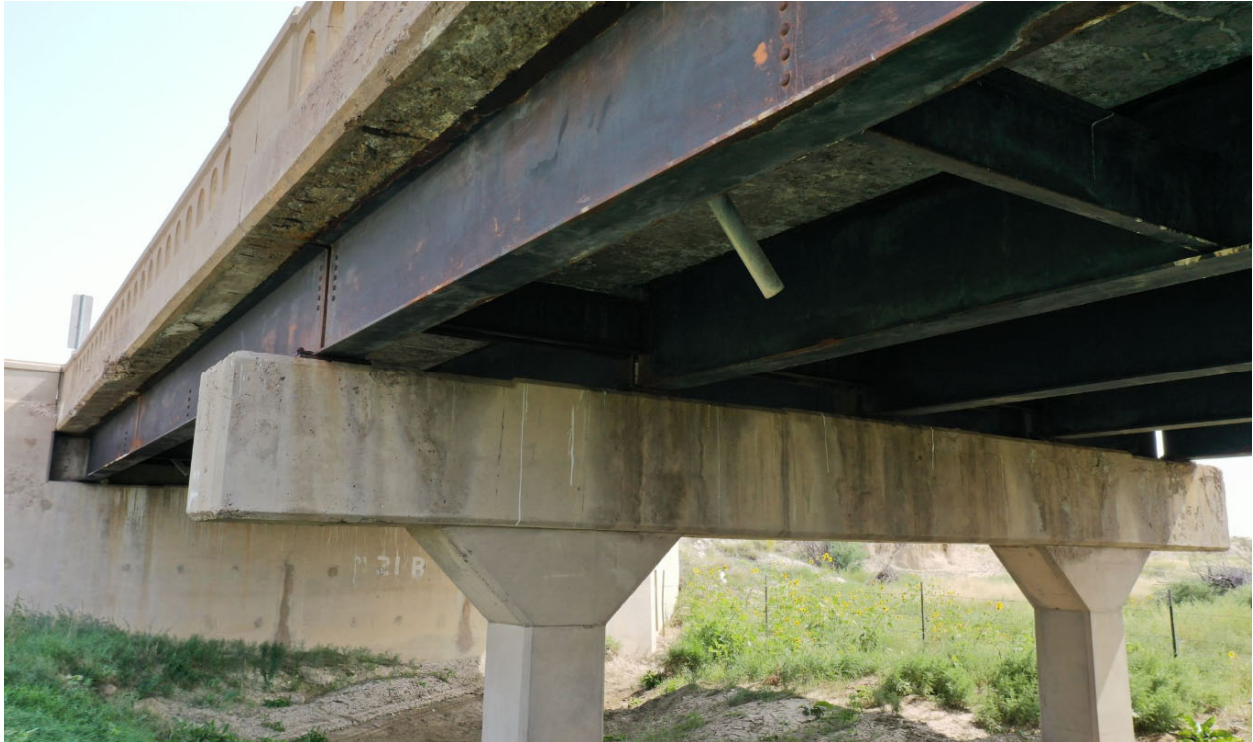
Picture 2 - Pier, Overhang, Deck, Girders
